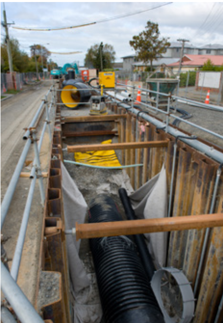
Wastewater pipe repairs on Edgware Road, St Albans.
