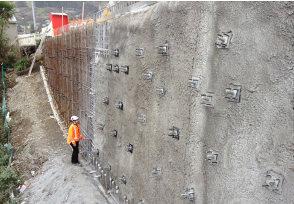
SCIRT engineer inspects the first layer of shotcrete on a Sumner Road retaining wall repair.
