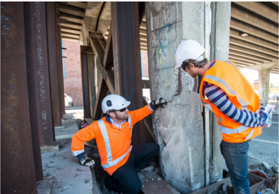
SCIRT project manager Phil Owen (crouching) and engineer Dean Bennett last year checking cracks to one of the piers of the Moorhouse Avenue overbridge.
