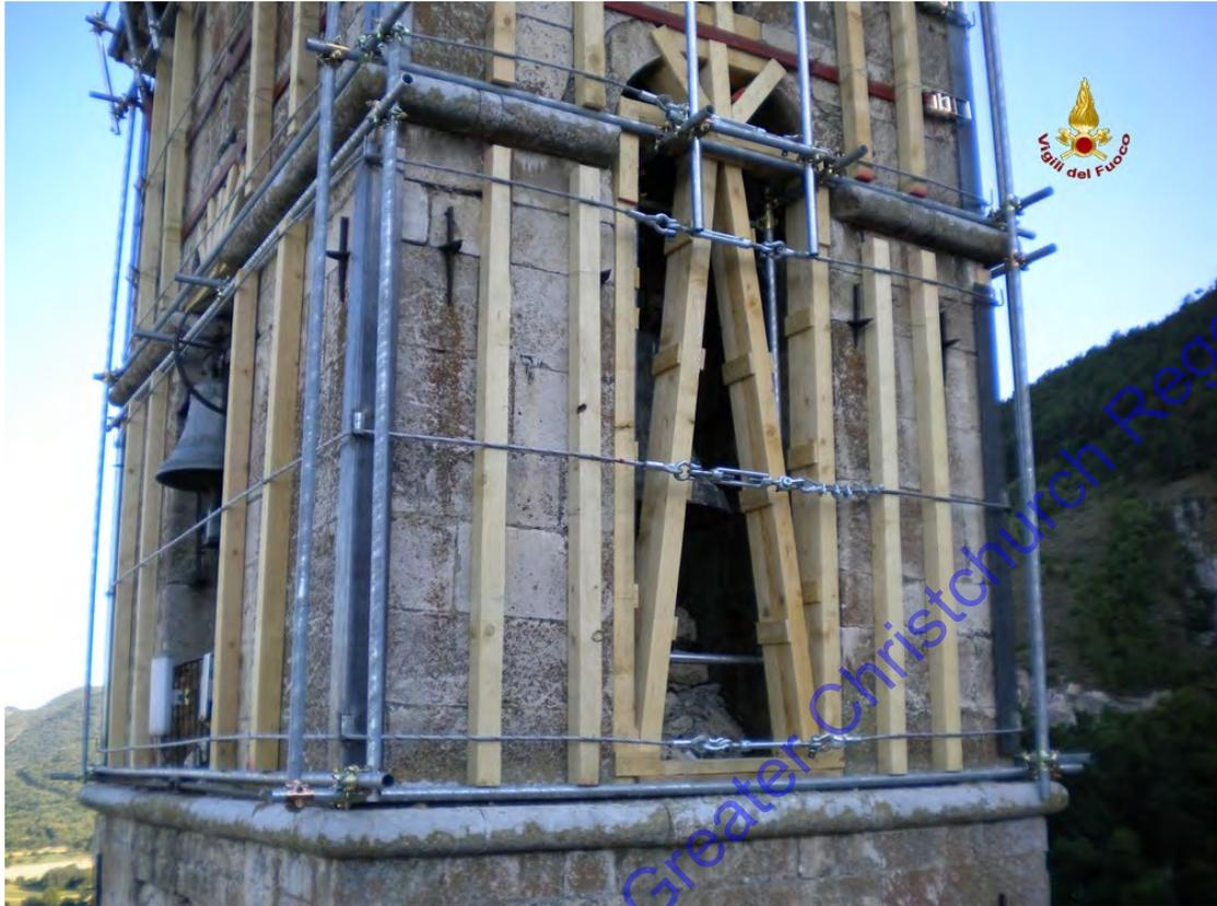
**Photograph 7: Tower clamped together with external perimeter ties, and openings strutted with timber framing.**
