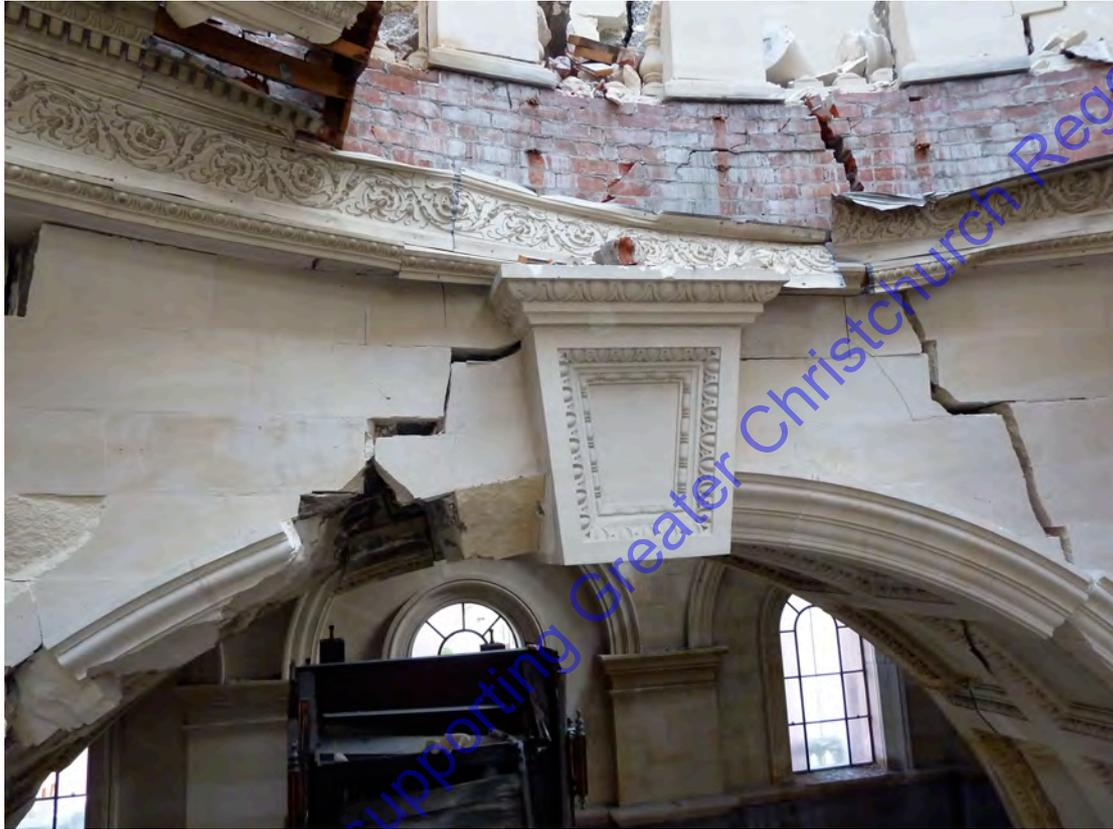
**Photograph 1: Christchurch Basilica, earthquake damage due to vertical shear-distortion up through the south arch forming the Crossing of the Nave and Transept. This distortion was due to the rocking in the east-west direction of the four columns supporting the four arches of the Crossing.**
