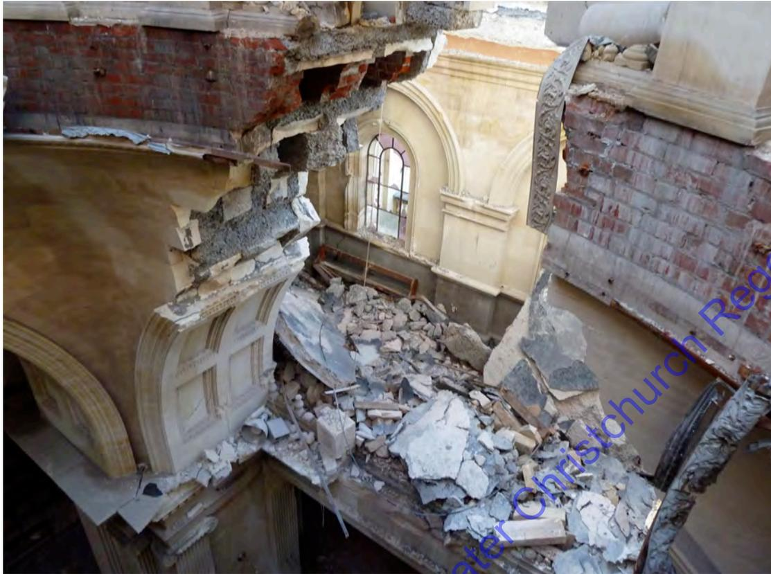
**Photograph 2: Christchurch Basilica, earthquake damage due to vertical shear-distortion up through the north arch forming the Crossing of the Nave and Transept. This distortion was due to the rocking in the east-west direction of the four columns supporting the four arches of the Crossing.
