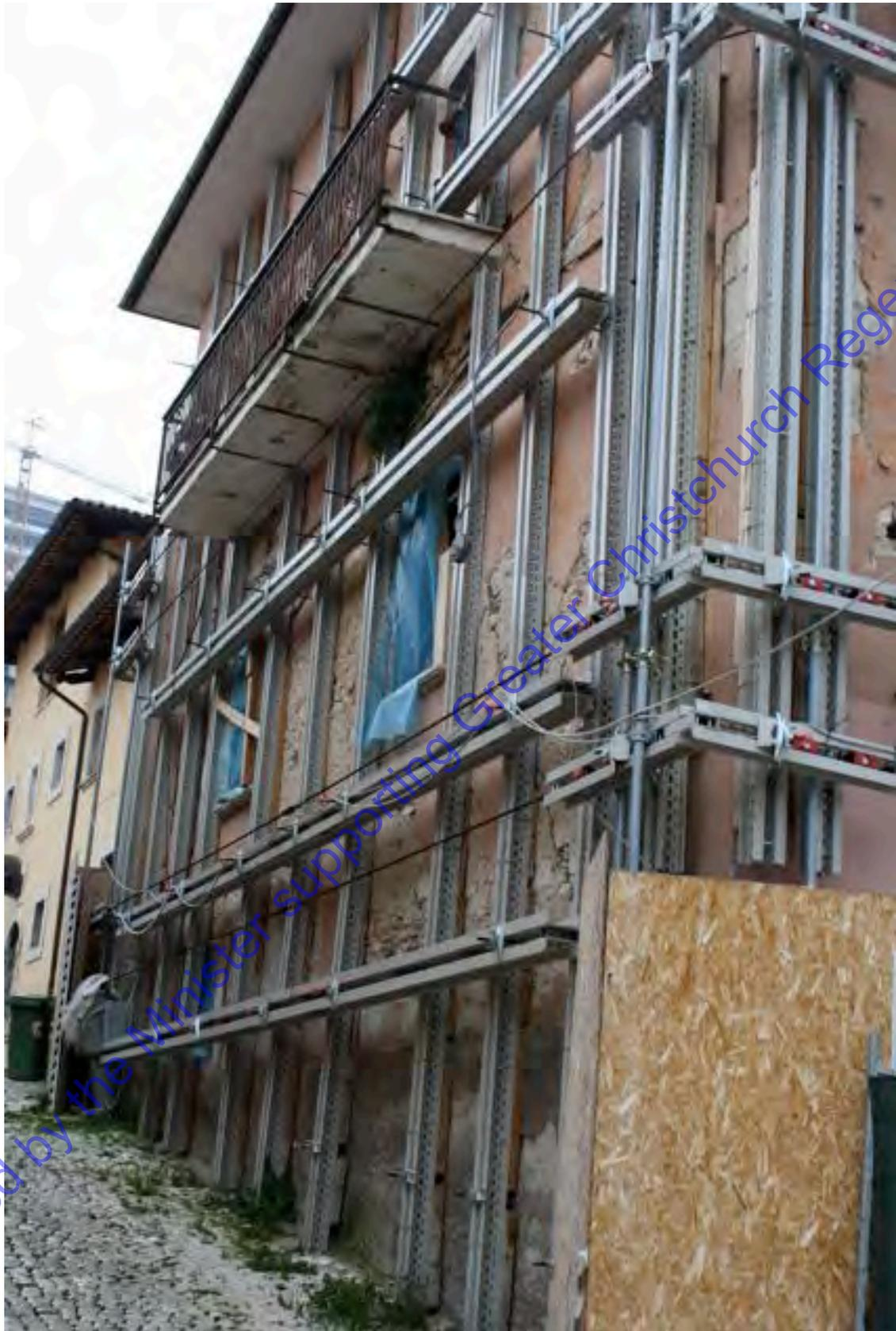
**Photograph 6: Ties through building to external frames to clamp masonry building together.**
