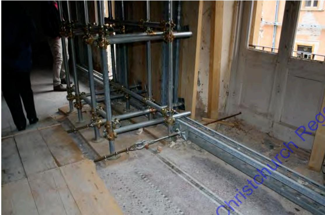
**Photograph 4: Masonry clamped between Inner and Outer tubular towers**
