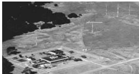
GCSB's radio communications interception station at Tangimoana, near Bulls.
