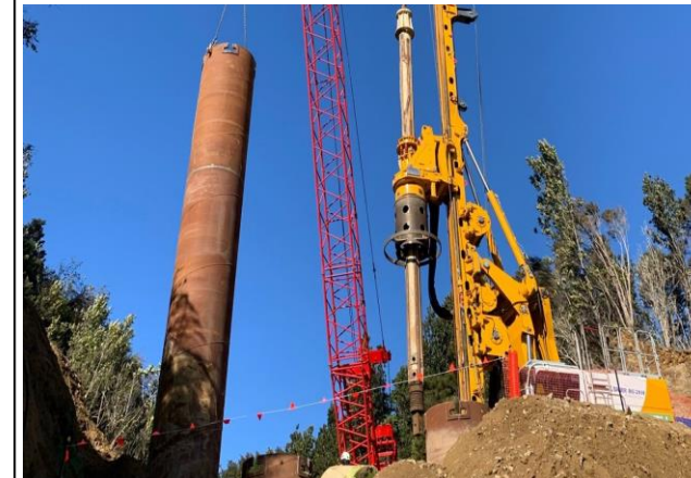
One of the piles for the Taparahi bridge on SH25A
