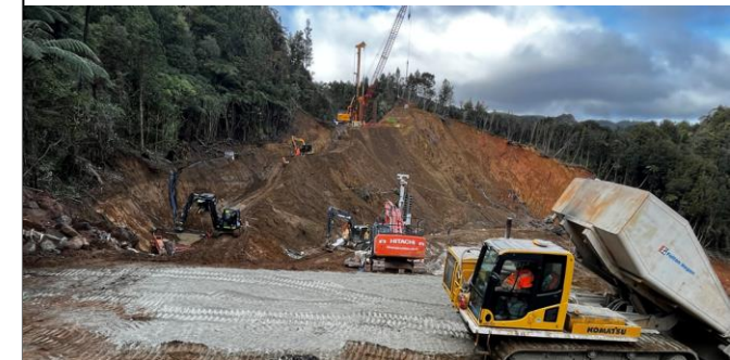
Construction of the Taparahi bridge on SH25A
