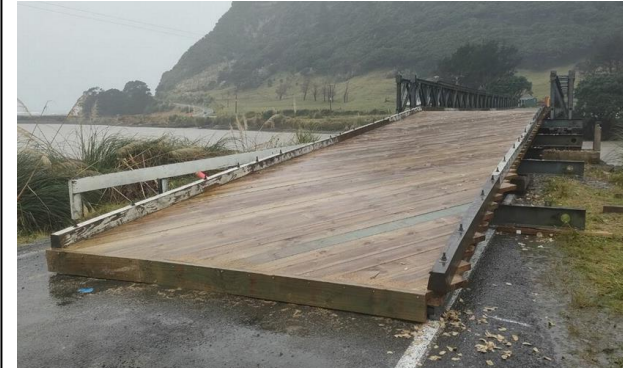
Awatere river bailey bridge. 21 July 2023 This bridge is now complete and open to traffic.
