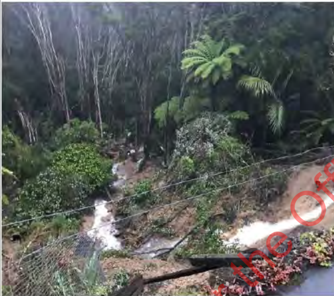
A slip in Titirangi that is impacting on water supply. Source: Watercare NZ Twitter
