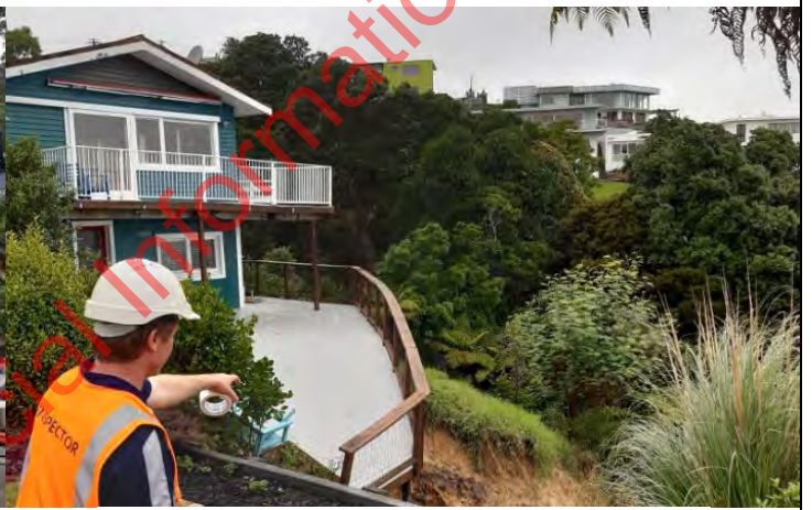
Building assessments taking place in Auckland Source: Auckland Emergency Management | Facebook
