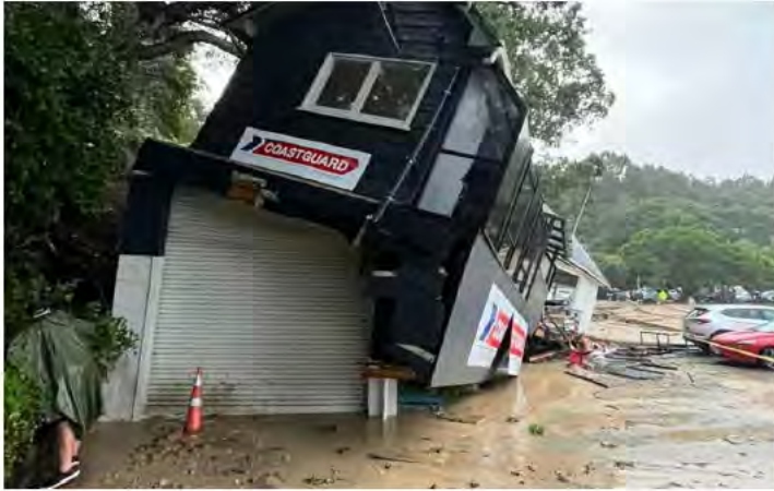
Land Slips brings down the Titirangi Coastguard building. Source: One News
