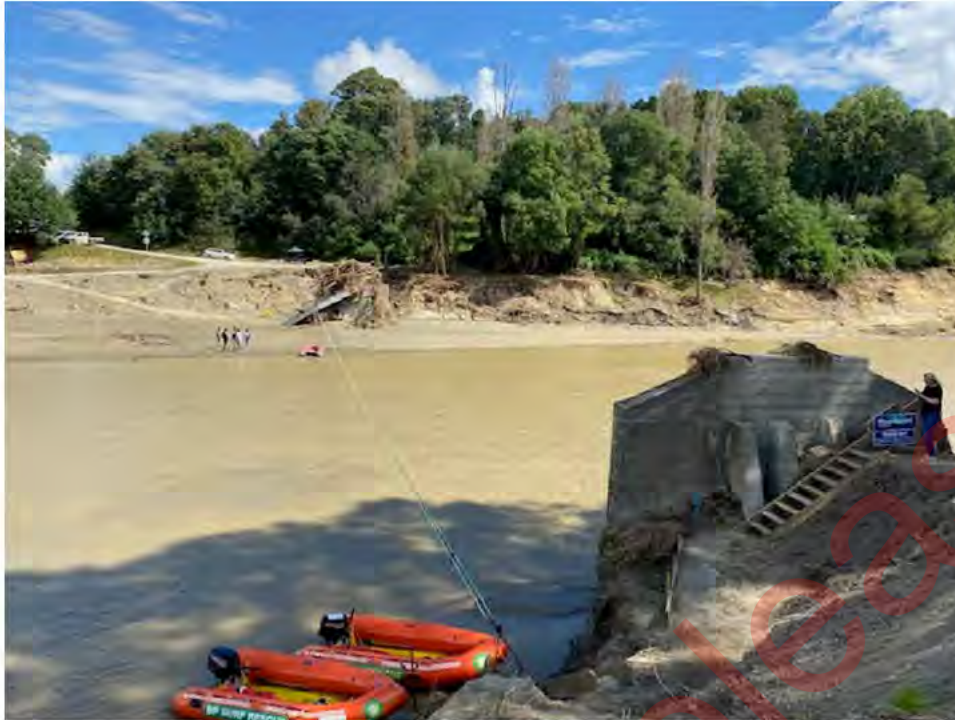
Figure 1: Rope pulley system and SLNZ IRBs at the Mangaone River crossing- Puketapu side of crossing
