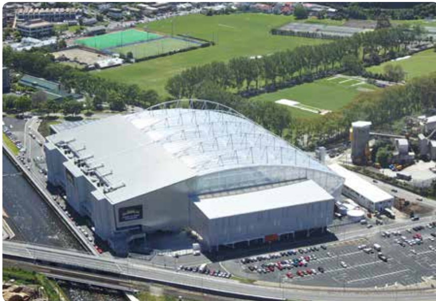
Forsyth Barr Stadium, Dunedin. Photographer: Darcy Schack, JAM Photographics Limited
