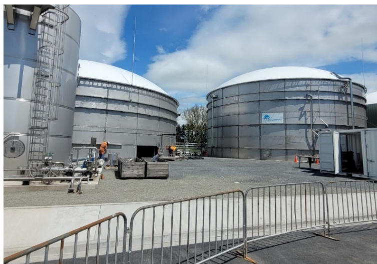
Figure 47: The digester tanks at Reporoa which hold up to 3.5 million litres of organic waste. Methane rises to the top of the tanks and are captured using a hose system.
